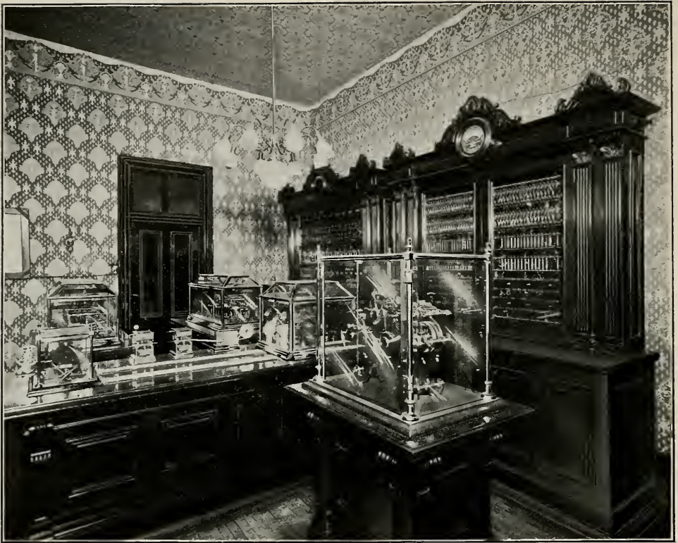
TRANSMITTER AND LINE-TESTING BOARD
